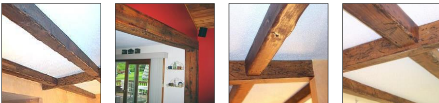
Box Beams & Casings
